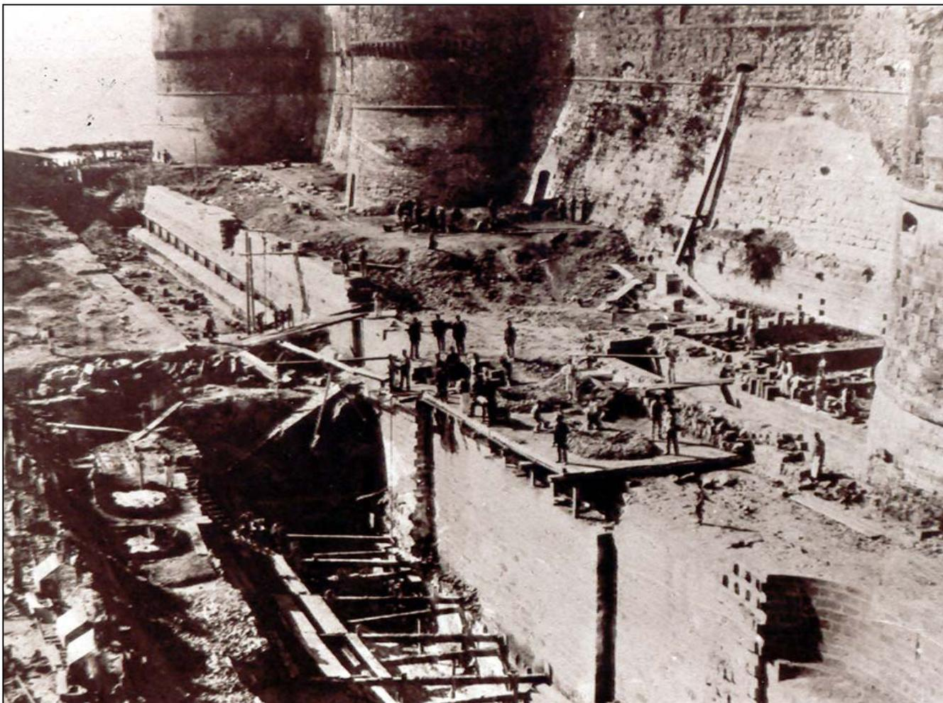
**Figure 3.4** – *The construction works of the navigable channel in a photo of 1885 (Mastronuzzi's Collection)*
